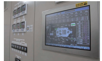
The operation panel enables manual operation as well as program operation in accordance with the standard.
