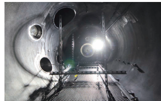
View from inside the tank where lighting, cameras, fuel spray nozzles, sensors, and so forth were installed.
